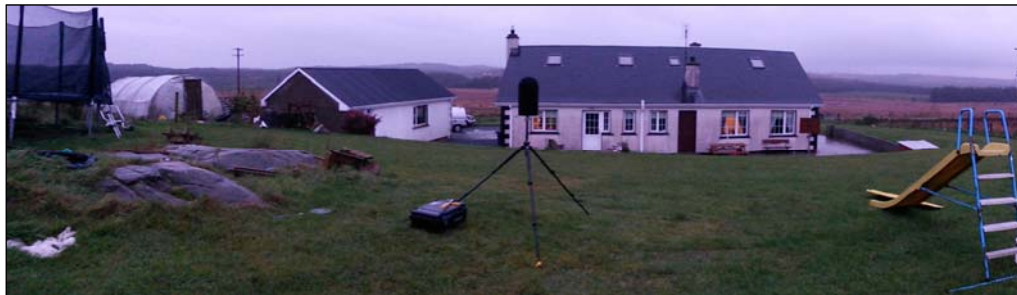
Figure 11.3 Location B (R255) Installation
