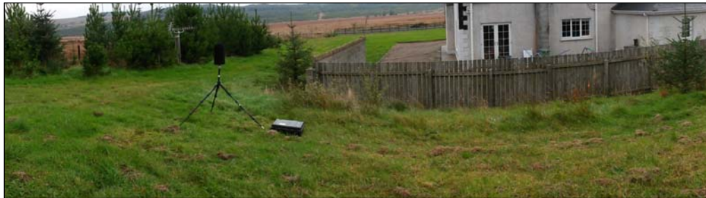
Figure 11.2 Location A (R256) Installation
